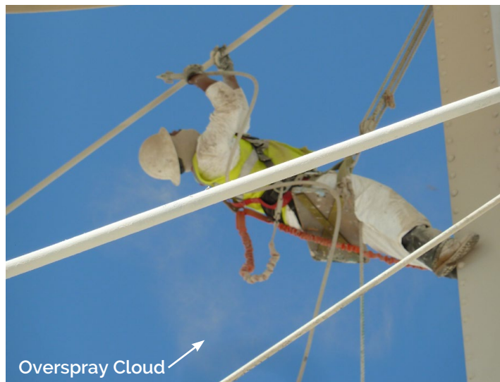
An overspray cloud can be seen around this painter.
